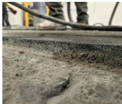
Mechanical removal and prep down to sound concrete.
