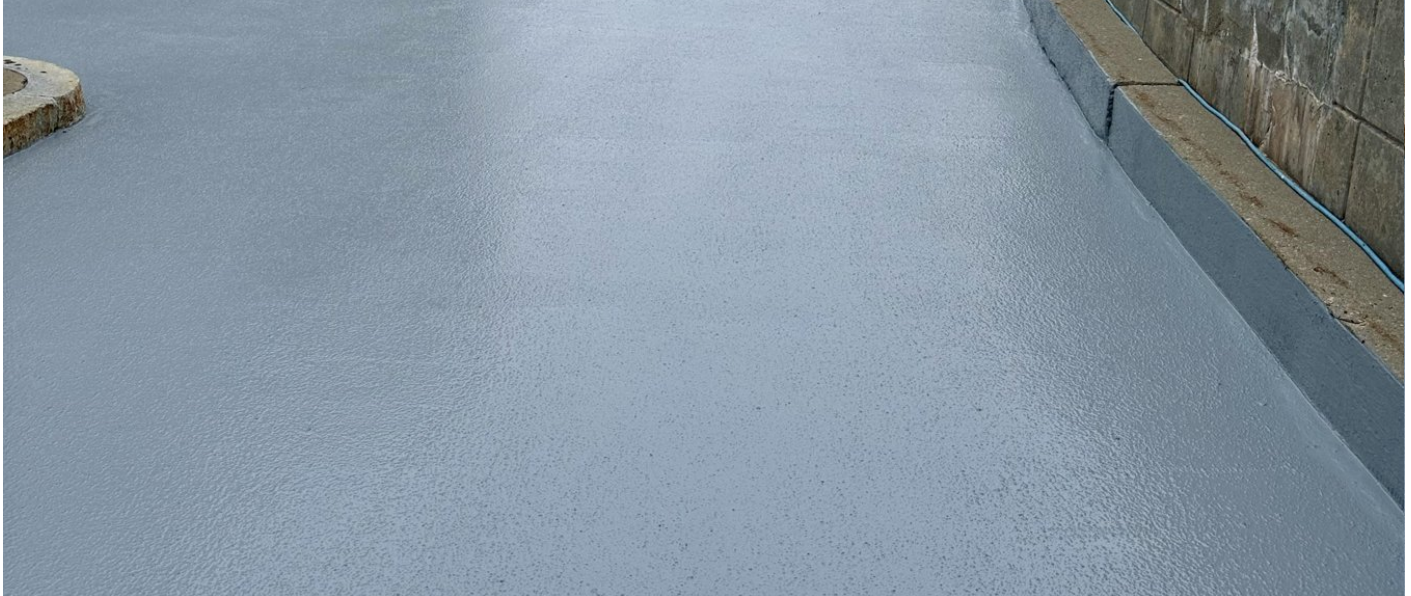
Polyurethane traffic coating on a vehicular ramp.
