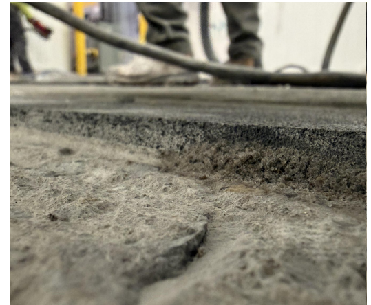
Diamond grinding with dust collection.
