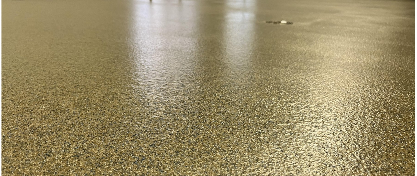
Decorative flake broadcast with a polyaspartic topcoat, commercial back-of-house.
