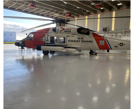
High-build epoxy in an aviation hangar.
