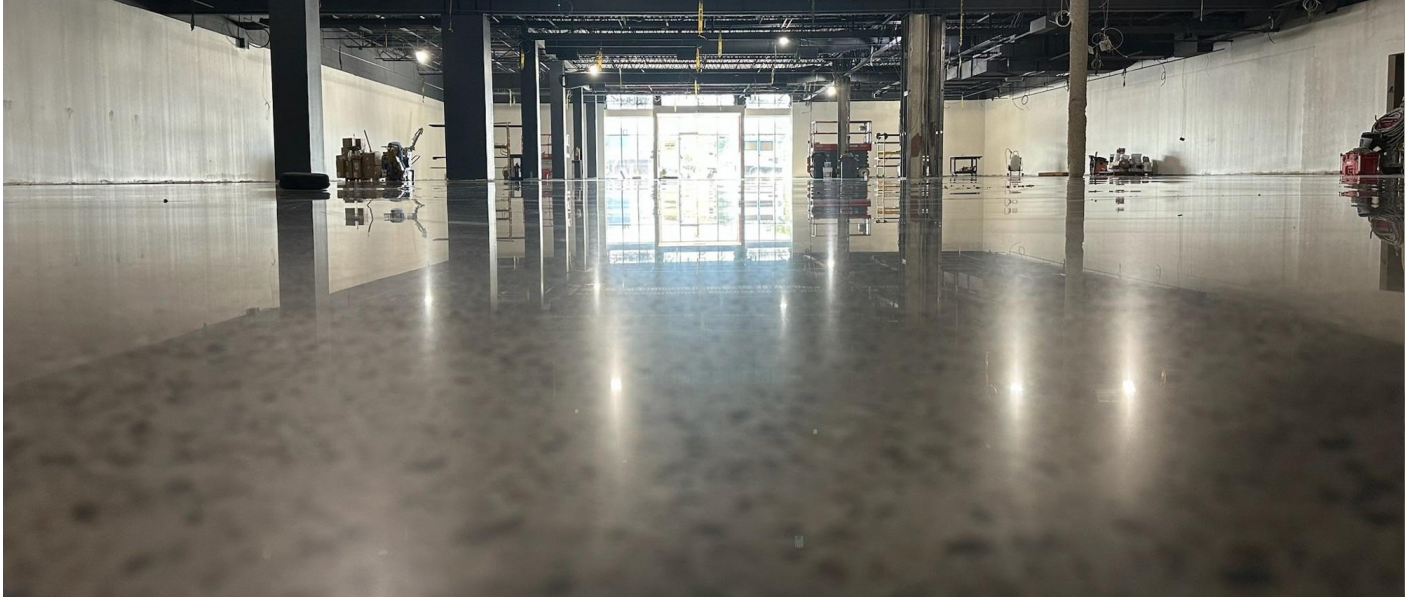
18,000 SF Class 3 polished floor, L.L. Bean Outlet, Framingham, MA. Other polishing contractors had classified this slab as not viable.
