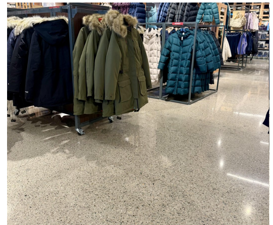
The Framingham floor after fit-out.
