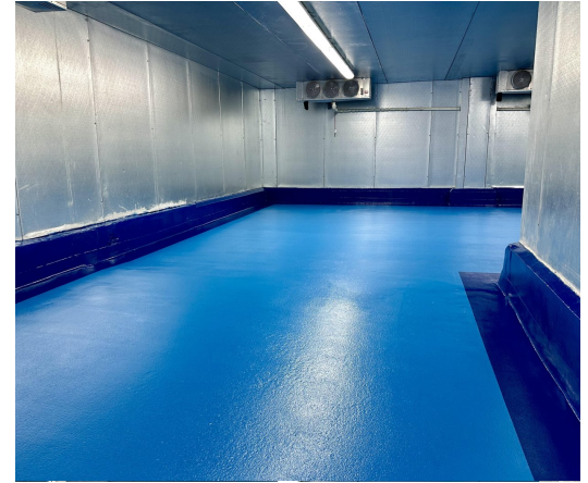
Urethane cement with integral cove, cold storage walk-in.
