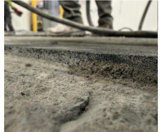
Slab prep before testing and install.
