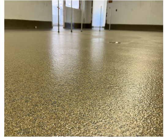
Flake broadcast with a polyaspartic topcoat.
