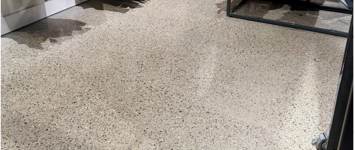
Class 3 polished concrete in service, L.L. Bean Outlet, Framingham, MA.
